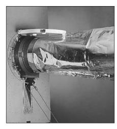
Pneumatic umbilicals are used for air conditioning of satellites with purified dry air during pre-launch phase. Disconnection is ensured by the vehicle.
